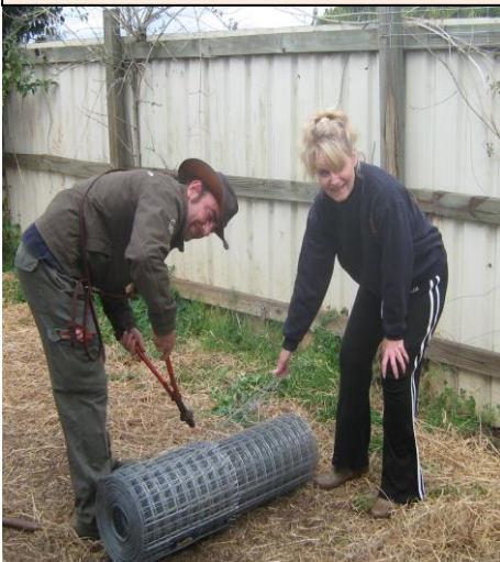
Suzanne and Luca doing some Fencing repairs at the centre
